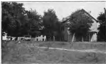
SOUTH CARROLLTON PUBLIC SCHOOL Formerly one of the West Kentucky College Buildings
